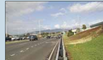
Moanalua Rd Freeway On-Ramp Lane Extension: Project extended an existing freeway onramp lane utilizing a paved shoulder to increase the storage of the lane. This resulted in more efficient operation of Moanalua Rd. New lane opened in Mar 2009.
